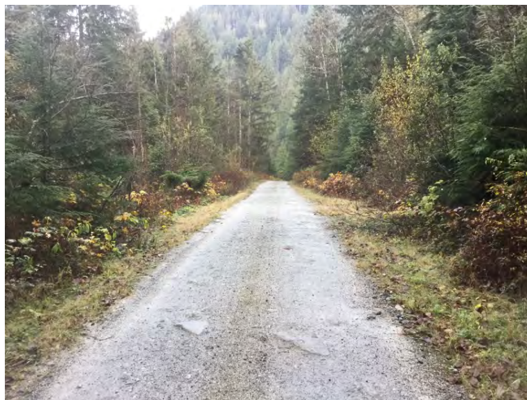
Approach from Left Bank when facing downstream
