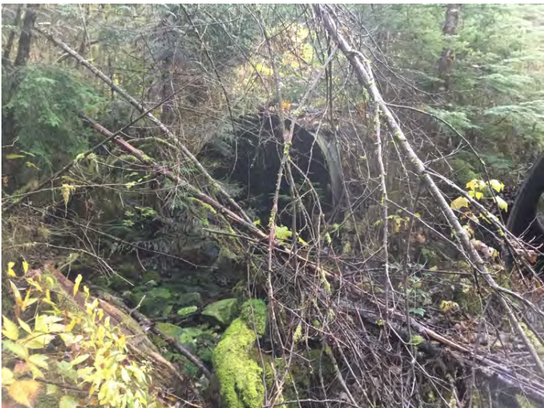
Outlet of 2000mm over flow culvert
